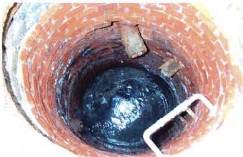
BRICK MANHOLE BEFORE REHABILITATION
