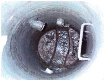
PERMACAST REHABILITATED MANHOLE
