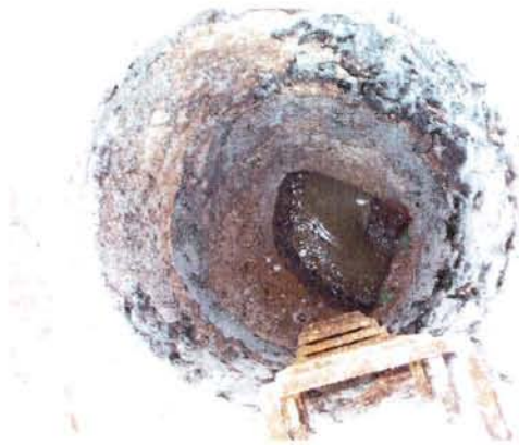
SEVERELY DETERIORATED CONCRETE MANHOLE
