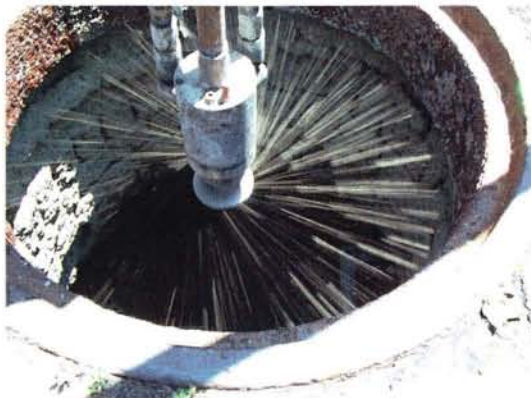
PNEUMATIC SPIN CAST APPLICATION OF REHABILITATION MORTAR
