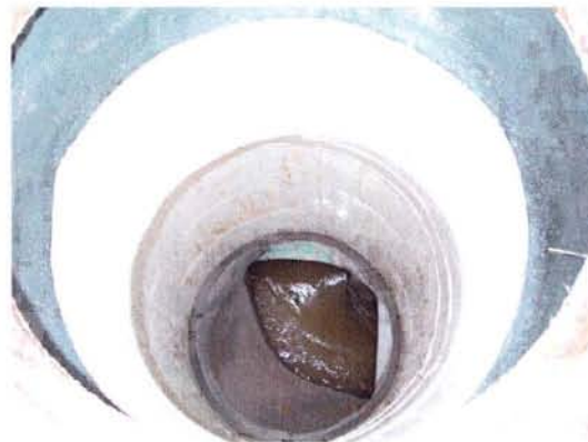
NEW 4" THICK CONCRETE MANHOLE IS FORMED AND- POURED WITH INTEGRATED T-LOCK PVC LINER
